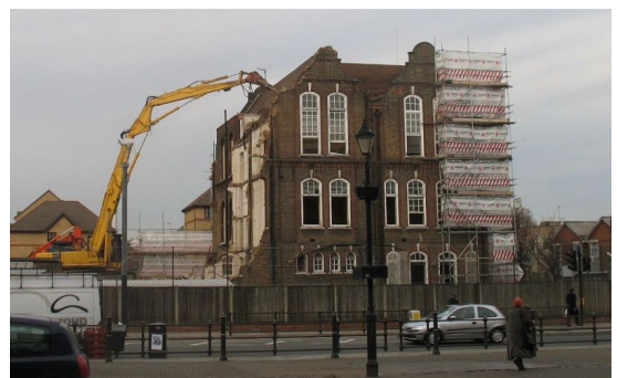
Bonners Street Primary School demolished 2007
